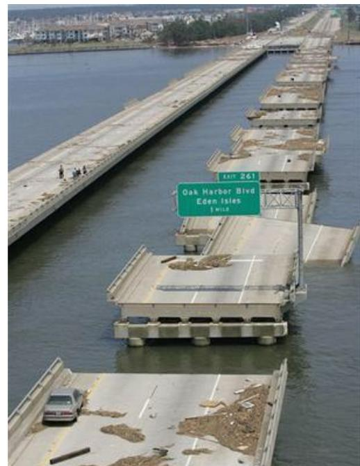
**Figure 1. Damage to the Twin Spans**
