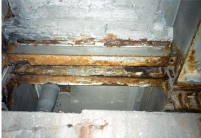
**Figure 4. Corrosion in Steel Beams**
